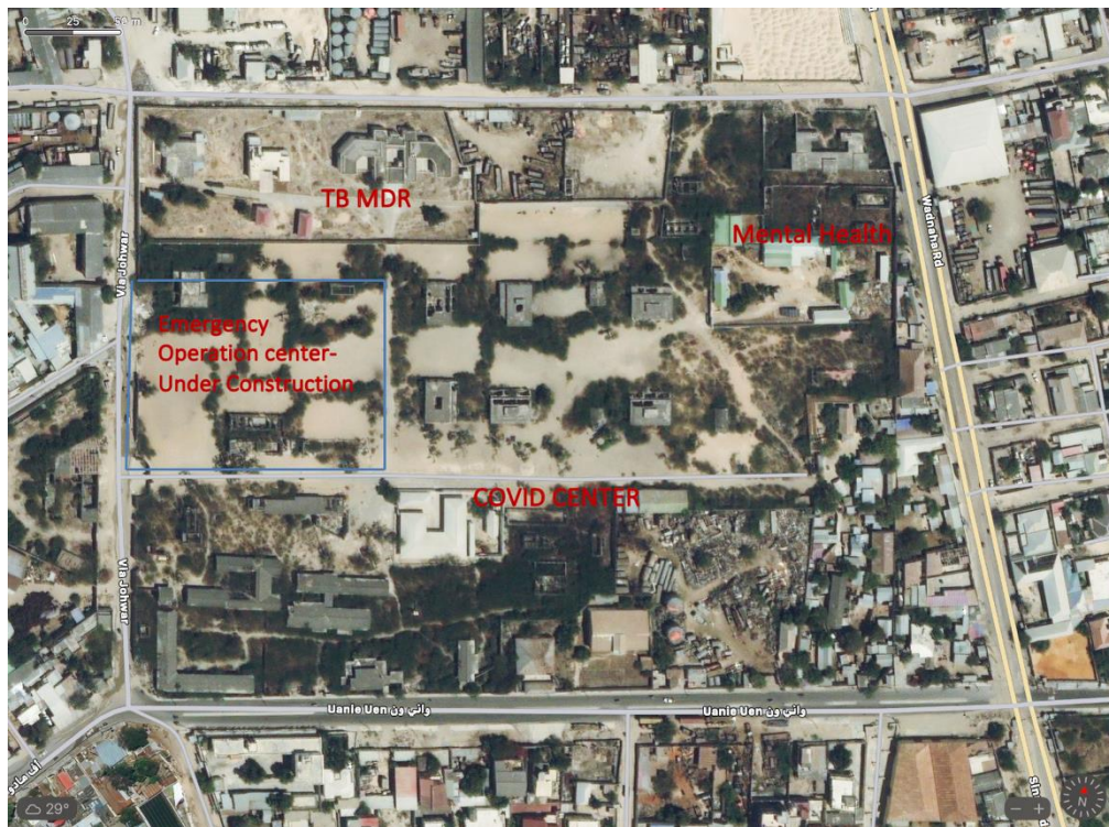
Figure 1: An aerial view of the hospital
