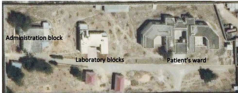
Figure 2: TB MDR Section aerial view
